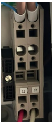
Figure 4.10 AC Connection Area of Inverter
